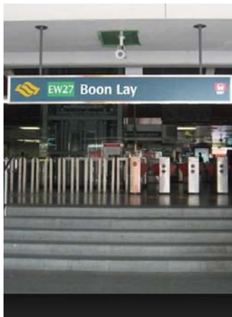
Boon Lay Station
